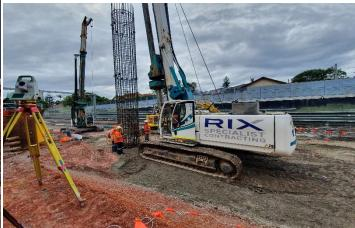
RIX was selected to undertake the piling works in the proximity to the live main north shore rail line at Chatswood Northern Dive in accordance with the relevant RMS specifications B59 & B80. This project was managed by Keshab SUBEDI
